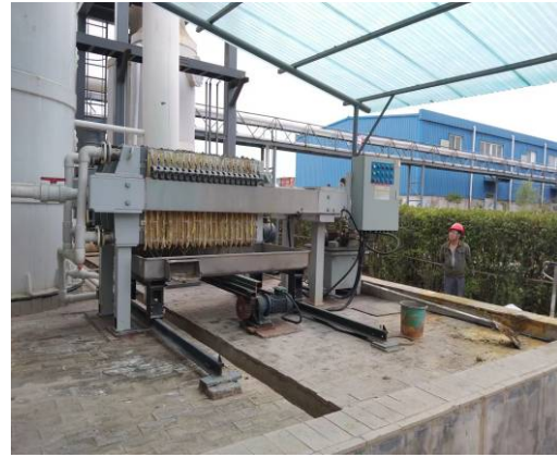
喷淋塔区围堰
